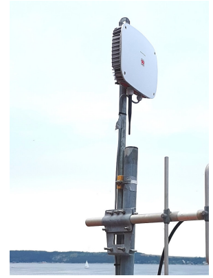
Fig. 2(c): Installed Shore Device
